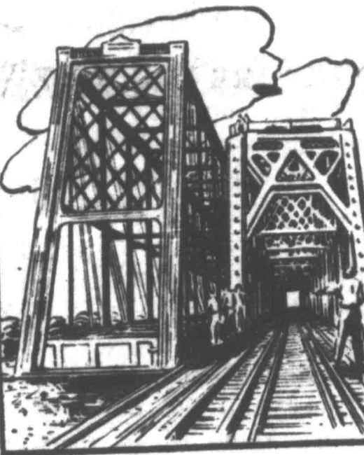
REBUILDING ITS BRIDGE ACROSS THE OHIO RIVER, A RAILROAD (1) MOVED AN OLD SPAN OFF ITS PIERS IN 57 MINUTES; (2) MOVED A NEW 518-FOOT SPAN TO THE SAME PIERS IN 75 MINUTES; (3) HOOKED UP THE TRACKS AND RESUMED FULL MAIN LINE OPERATIONS ALL WITHIN 20 HOURS.
